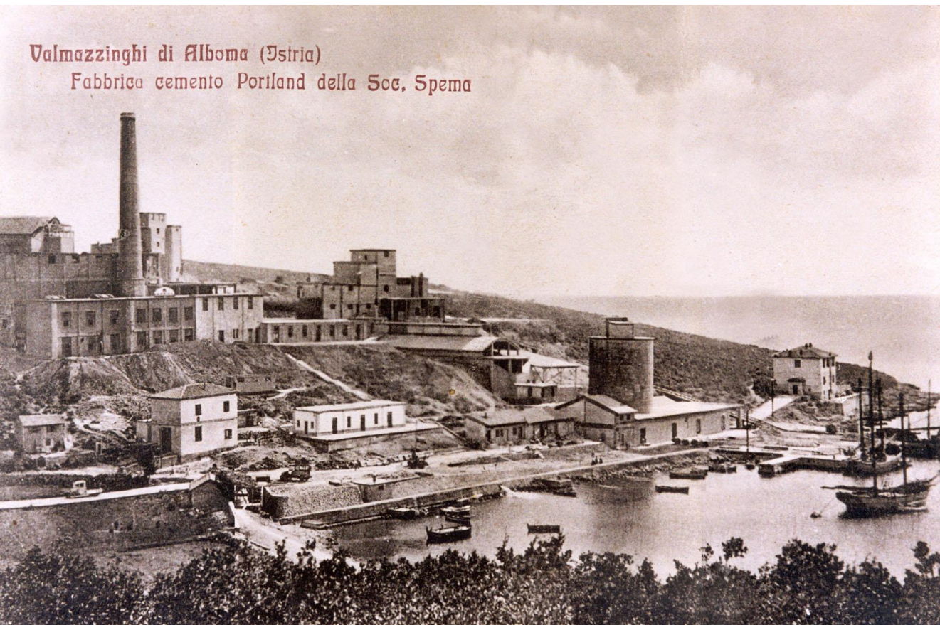
1926 - Start of cement production in Koromačno
